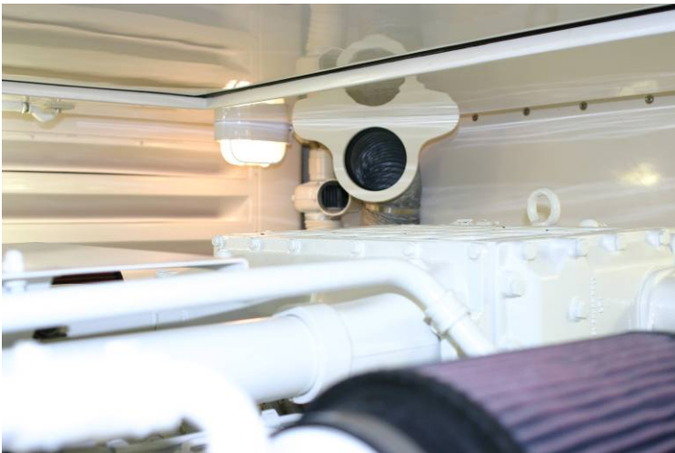
Ref# 301 A/C ENGINE ROOM
